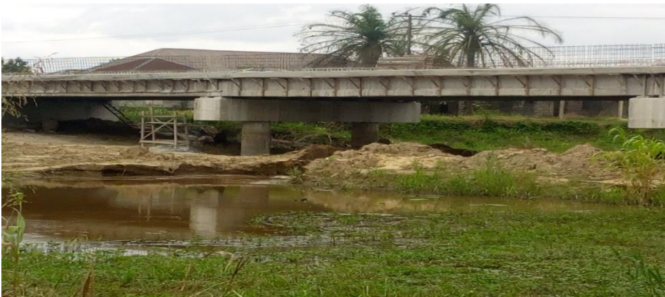
Plate 2. Ongoing Bridge Constructions in the Kolo Creek
